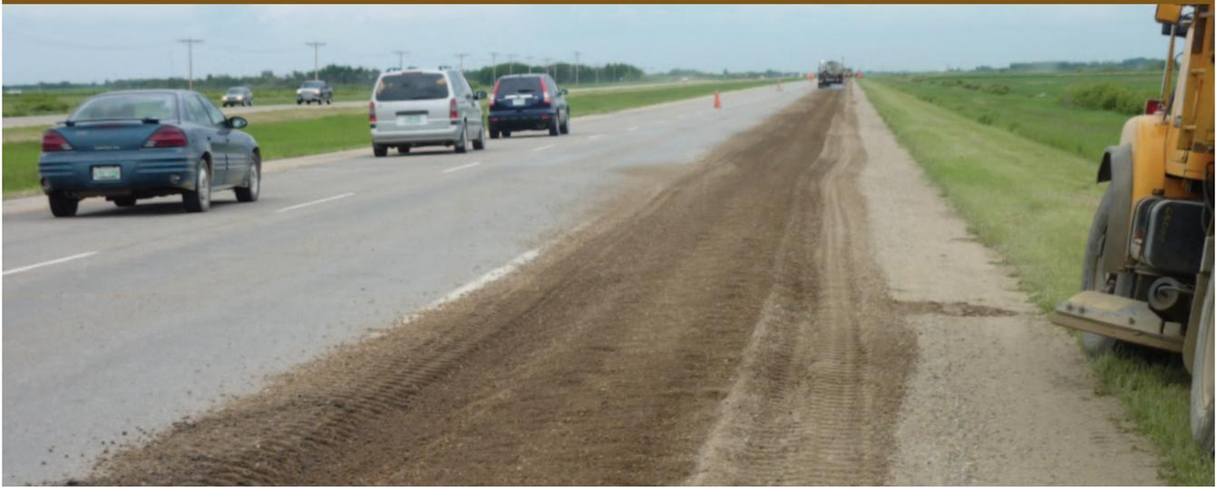
**Project Description:** Terratech polymer technology was used for road shoulder stabilization along Highway 16 near Saskatoon, Canada. A 1.5 m wide section of road shoulder was stabilized intermittently between asphalted sections. Vehicular wear and shoving of the aggregate from the surface caused deterioration of the shoulder and a potentially hazardous condition for trucks and cars.
